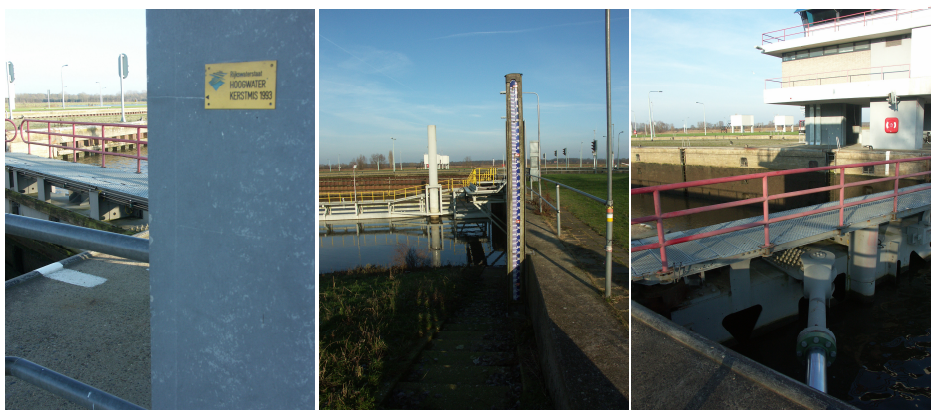
Figure 2.6: Weir at Sambeek; the yellow plaque indicates the maximum 1993 water levels (left) at ~13.70 m above sea level. In these pictures, water levels are c. 11.7m above sea level. Sambeek is located close to rkm 150 (see e.g. Figure 2.7).
